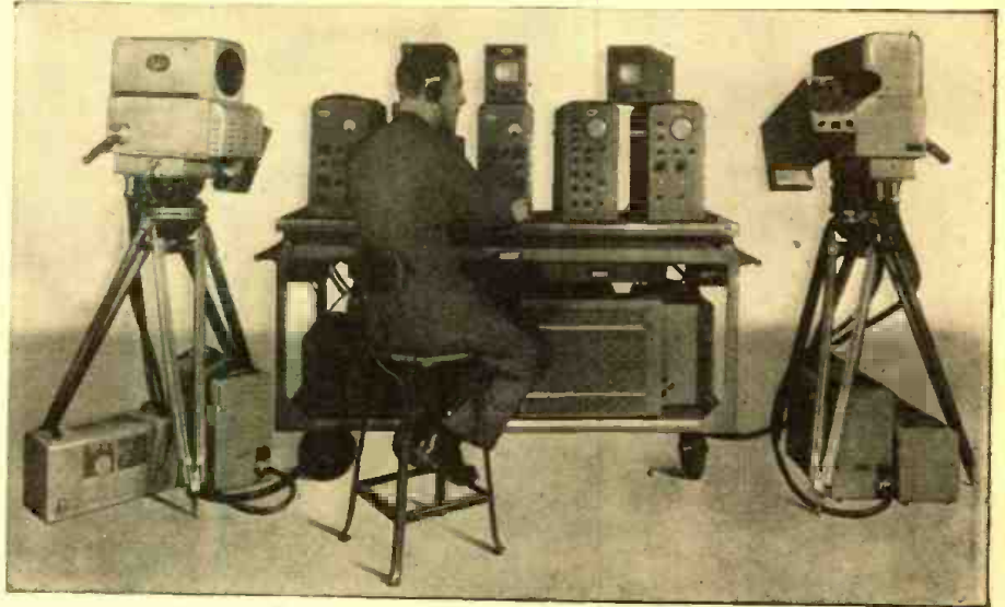
Engineer at lineup of unit television setup. See text for details.
